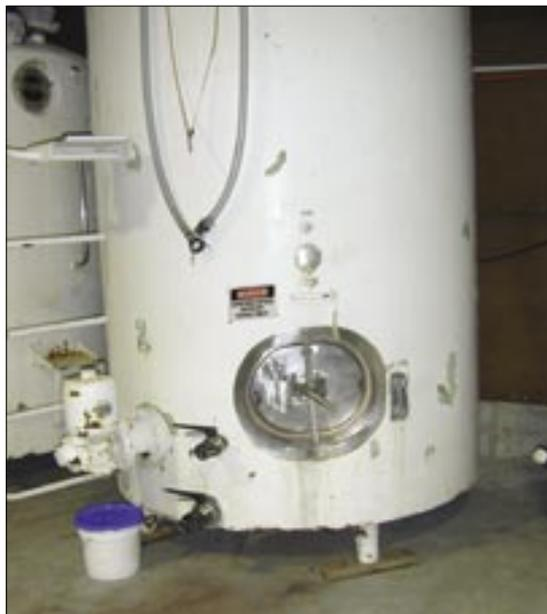
*A vat is a confined space in your workplace. If the material inside is fermenting, there might not be enough oxygen for you to breathe, or carbon dioxide may be present in toxic amounts. Either condition can cause you to collapse. If cleaning or welding is being done inside a confined space such as this one, hazardous gases might be produced. Before anyone enters a confined space, the space must be made safe to enter. Safety precautions include testing the atmosphere and ventilation.*
